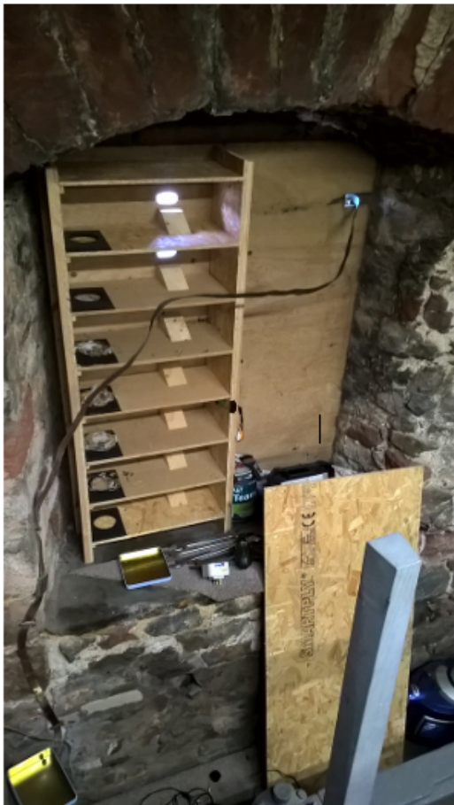
Kingsteignton church boxes installed in 2018. The ramps were installed to help the swifts leave the box as the hole was quite high from the floor. A bell stay is visible lower right.
